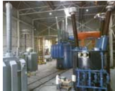
View of test bay
